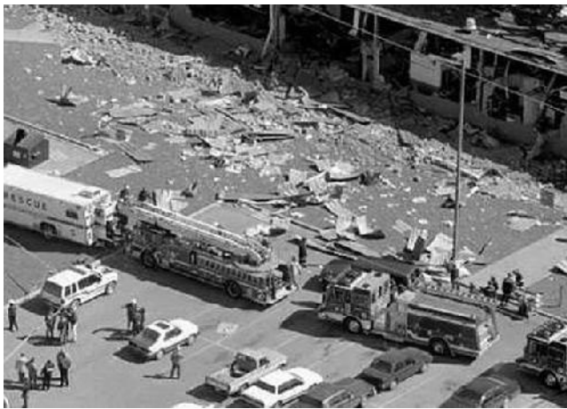
Figure 2 : Overview of the Molding workshop devastated by the explosion, photograph 60 hours after the incident
